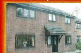
PVC Door & window canopies supplied and fitted
