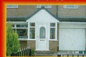
Replaced or built from scratch
