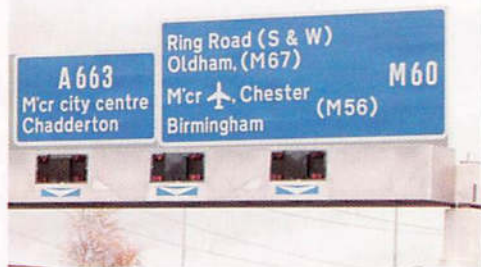
The M60 Motorway
